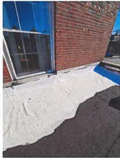
Area of repair previously done
