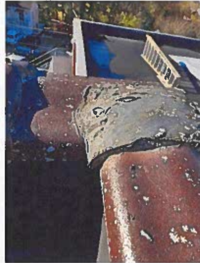
Repair on parapet cap for Front Upper Roof
