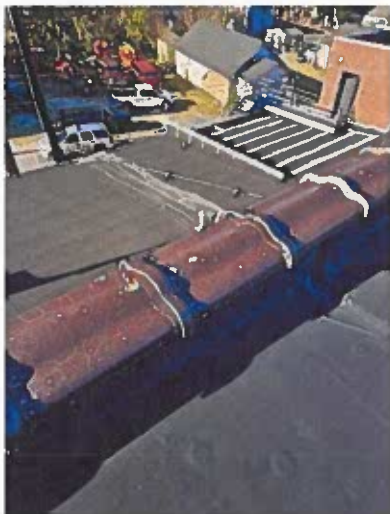
Overview of the lower front roof
