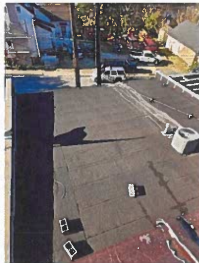
Overview of rolled roofing covering the lower front roof
