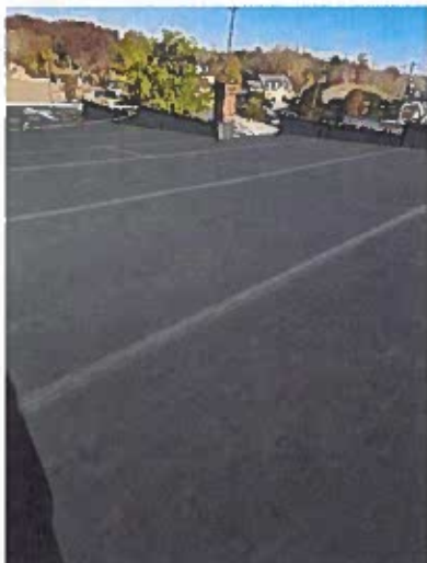
Overview of the front upper roof
