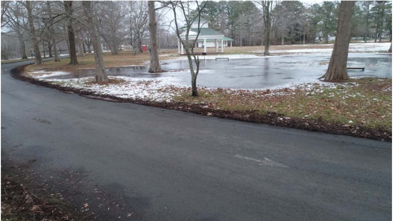
IMAGE 3: DOCUMENTED PONDING/FLOODING IN JANUARY 2022
